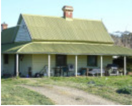
190879_Emu Creek_Hargreaves Road_148_img01
