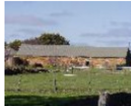
192577_Emu Creek_Red Tank Road_197_img08
