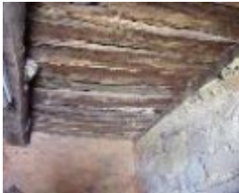
192577_Emu Creek_Red Tank Road_197_img11
