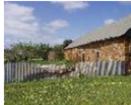
192577_Emu Creek_Red Tank Road_197_img07
