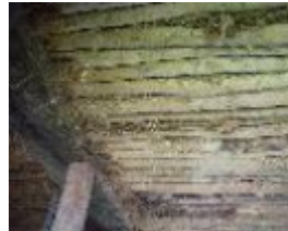
192577_Emu Creek_Red Tank Road_197_img10
