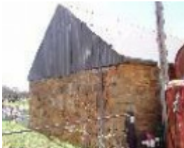
192577_Emu Creek_Red Tank Road_197_img05
