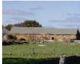
192577_Emu Creek_Red Tank Road_197_img08
