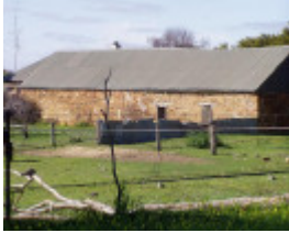
192577_Emu Creek_Red Tank Road_197_img01
