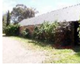
192577_Emu Creek_Red Tank Road_197_img03
