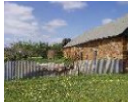
192577_Emu Creek_Red Tank Road_197_img07
