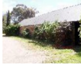
192577_Emu Creek_Red Tank Road_197_img03
