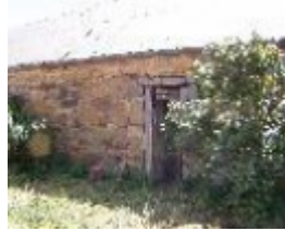
192577_Emu Creek_Red Tank Road_197_img04
