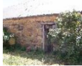
192577_Emu Creek_Red Tank Road_197_img04
