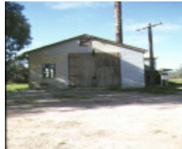
lock nine pumping station cullulleraine front view
