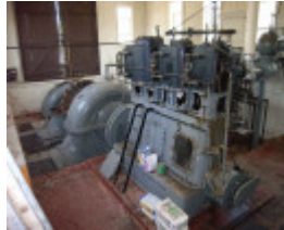
LOCK NINE PUMPING STATION SOHE 2008
