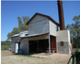
LOCK NINE PUMPING STATION SOHE 2008
