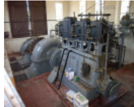
LOCK NINE PUMPING STATION SOHE 2008
