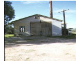
lock nine pumping station cullulleraine front view
