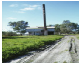
lock nine pumping station cullulleraine chimney view
