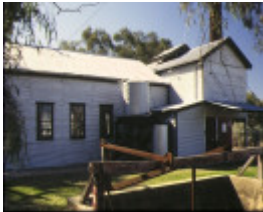
1 lock nine pumping station cullulleraine rear view oct1994
