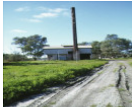
lock nine pumping station cullulleraine chimney view
