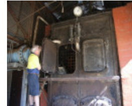
LOCK NINE PUMPING STATION SOHE 2008
