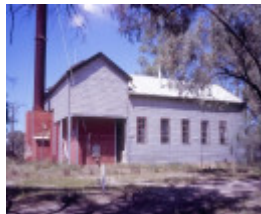
h00549 lock nine pumping station cullulleraine front riverside she project 2004
