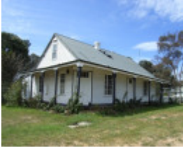
203611_Heathcote_Northern Highway South_6360_img01
