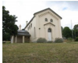
Court house front view. Feb 2008.
