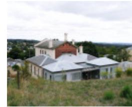
COURT HOUSE, FORMER POLICE QUARTERS AND LOCK-UP SOHE 2008
