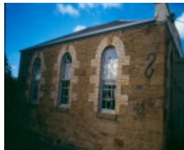
H02010 former weslyan chapel box hill west side
