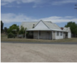
216164_Knowsley_Knowsley- Eppalock Road_011_img01
