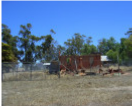
205904_Derrinal_Sheedys Lane_Murrowood Homestead_img01
