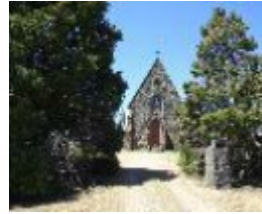
206149_Redesdale_Heathcote Redesdale Road_2115_img03
