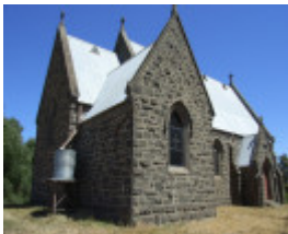
206149_Redesdale_Heathcote Redesdale Road_2115_img04
