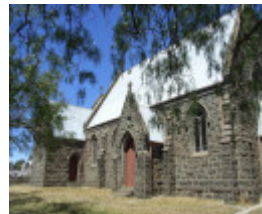
206149_Redesdale_Heathcote Redesdale Road_2115_img08
