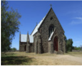
206149_Redesdale_Heathcote Redesdale Road_2115_img01
