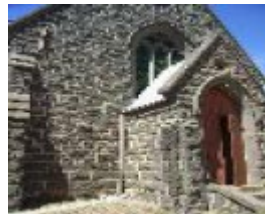
206149_Redesdale_Heathcote Redesdale Road_2115_img07
