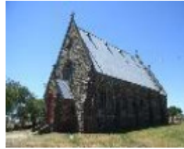
206149_Redesdale_Heathcote Redesdale Road_2115_img09
