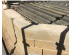
During Photograph - Reference F3890 2015
