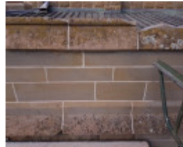
Before Photograph - Reference F3890 2014
