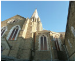
Before Photograph - Reference F3890 2014
