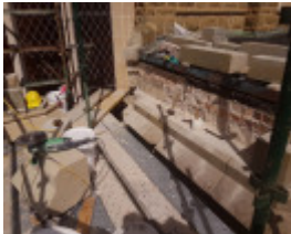
During Photograph - Reference F3890 2015
