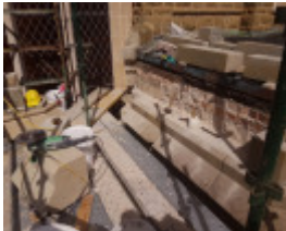
During Photograph - Reference F3890 2015
