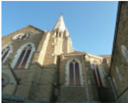
Before Photograph - Reference F3890 2014
