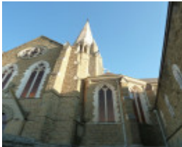
Before Photograph - Reference F3890 2014
