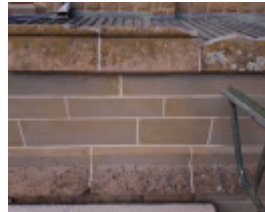
Before Photograph - Reference F3890 2014
