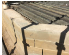
During Photograph - Reference F3890 2015
