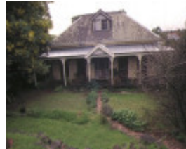
1 prefabricated residence ormond road moonee ponds front view
