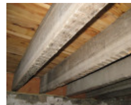
Ground floor from below
