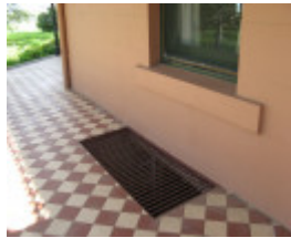
Mt Ridley homestead grill in verandah floor to light cellar
