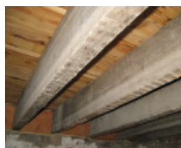
Ground floor from below
