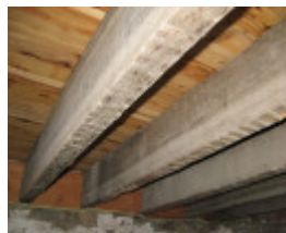
Ground floor from below
