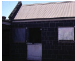
stables 1875 lara homestead derrinallum entrance
