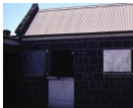
stables 1875 lara homestead derrinallum entrance
