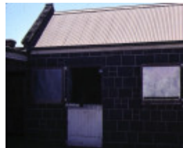
stables 1875 lara homestead derrinallum entrance
