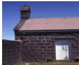
stables 1875 lara homestead derrinallum side view
