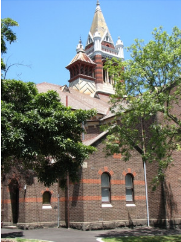
AUBURN UNITING CHURCH COMPLEX SOHE 2008
