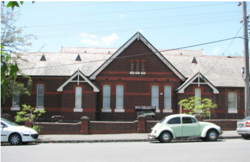
AUBURN UNITING CHURCH COMPLEX SOHE 2008
