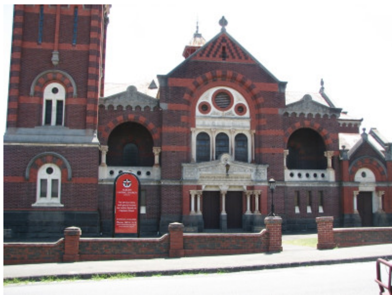
AUBURN UNITING CHURCH COMPLEX SOHE 2008
