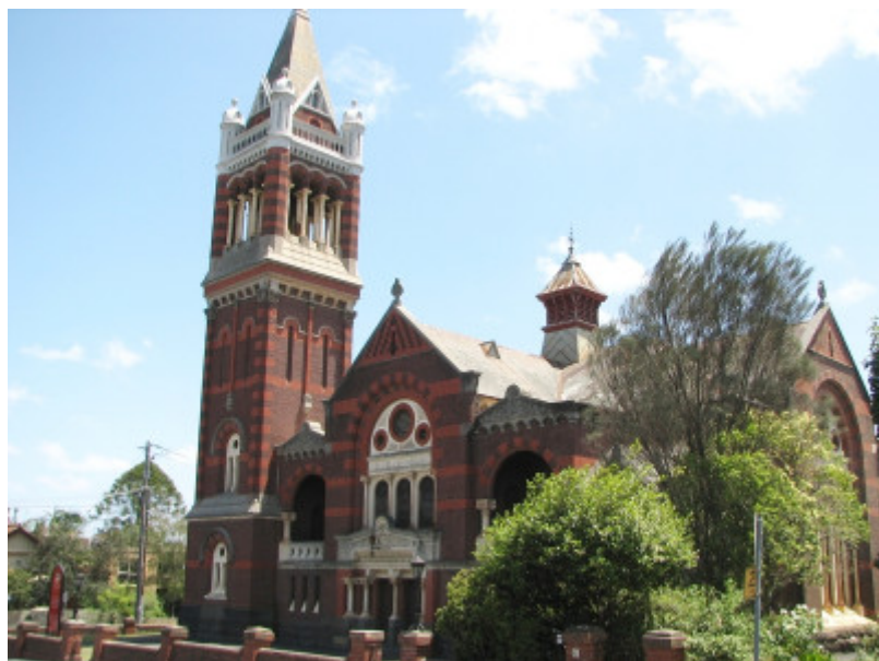
AUBURN UNITING CHURCH COMPLEX SOHE 2008
