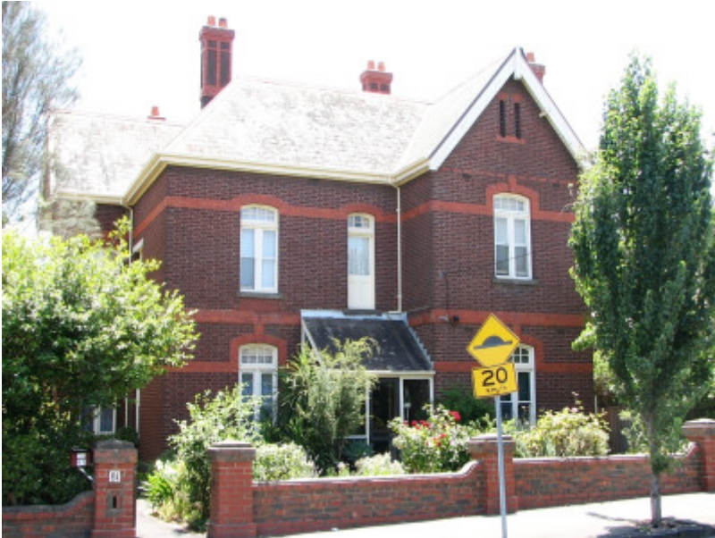
AUBURN UNITING CHURCH COMPLEX SOHE 2008
