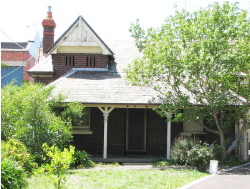
AUBURN UNITING CHURCH COMPLEX SOHE 2008
