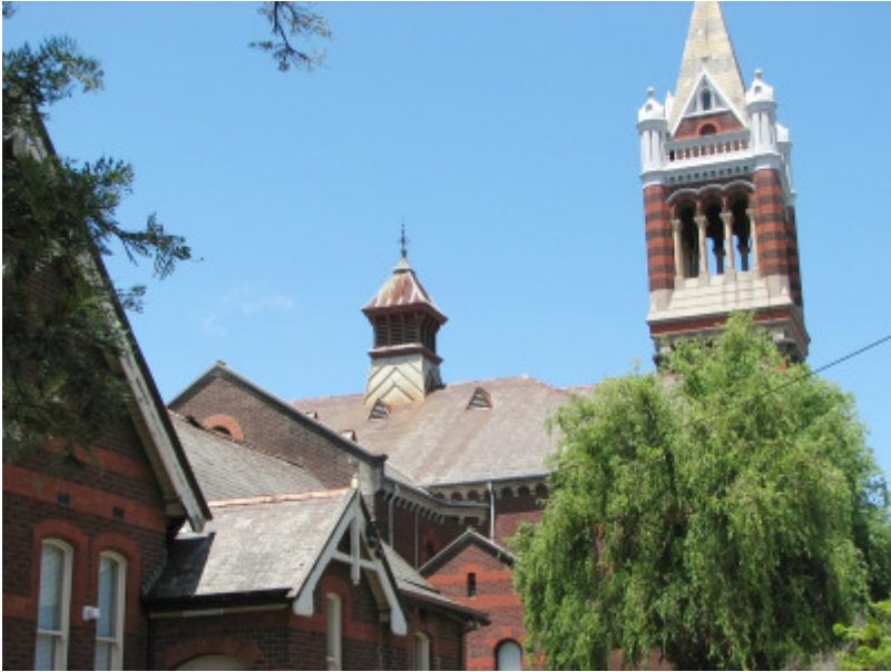
AUBURN UNITING CHURCH COMPLEX SOHE 2008
