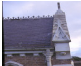
christ church old dandenong road dingley village roof view
