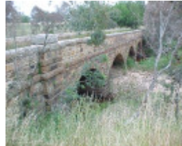
1 bridge over hughes creek avenel nov 99
