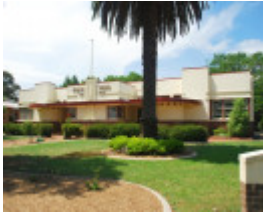
PRIMARY SCHOOL NO. 1924 SOHE 2008
