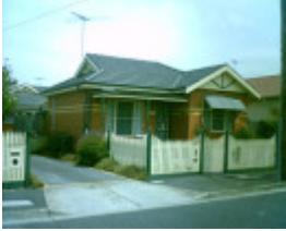
37 Catherine Street, Geelong West - Units
