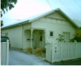
49 Catherine Street, Geelong West
