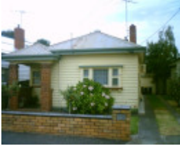
52 Catherine Street, Geelong West
