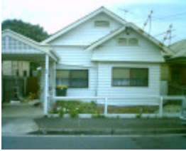
54 Catherine Street, Geelong West
