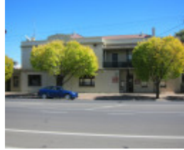
143 Charleston Road, Fleece Inn, detail of front verandah
