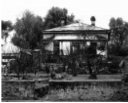
House at 257 Eaglehawk Rd
