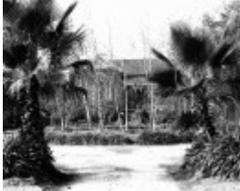
House at 6 Jennings St, East Bendigo
