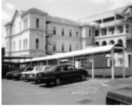
Bendigo Goldfields Hospital, Lucan Street
