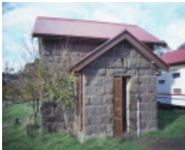
1 lock up parker street dunkeld entrance jun1984
