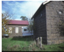
lock up parker street dunkeld side elevation jun1984
