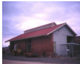
dunolly railway station goods shed may1995
