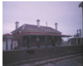
1 dunolly railway station trackside view may1995
