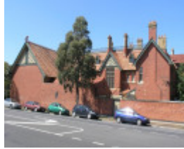
FORMER NORTH PARK SOHE 2008
