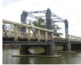
Barham Koondrook Bridge_Koondrook_Feb 2007_mz_Centre Lift Span
