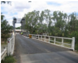
Tooleybuc Bridge_Piangil_Feb 2008_mz_Victorian Approach
