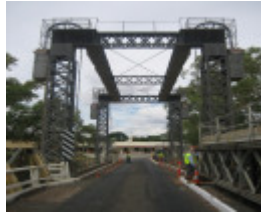
Tooleybuc Bridge_Piangil_Feb 2008_mz_Central Lift Span
