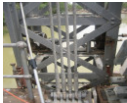
Tooleybuc Bridge_Piangil_Feb 2008_mz_Winch Detail
