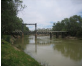
Tooleybuc Bridge_Piangil_Feb 2008_mz_West Elevation
