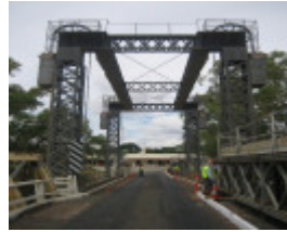
Tooleybuc Bridge_Piangil_Feb 2008_mz_Central Lift Span
