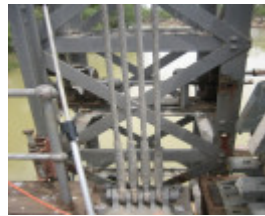
Tooleybuc Bridge_Piangil_Feb 2008_mz_Winch Detail
