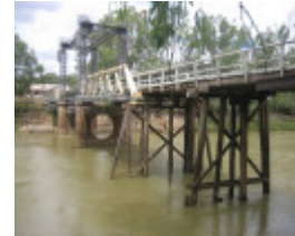
Tooleybuc Bridge_Piangil_Feb 2008_mz_Victorian Approach Spans
