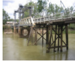
Tooleybuc Bridge_Piangil_Feb 2008_mz_Victorian Approach Spans
