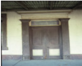
former bendigo hotel dunolly front entrance
