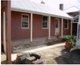
H2169 RIMG0148 - c.1849 cottage, 15-19 Gawler street, portland
