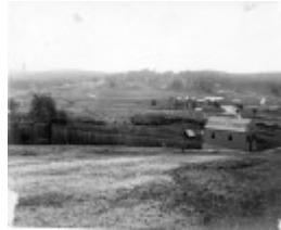
Grenville Standard Building, Linton and outlying township area, June 1909. Source: Linton Historical Society.
