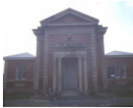
1 dunolly court house front elevation aug1984
