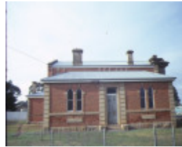
dunolly court house rear elevation aug1984
