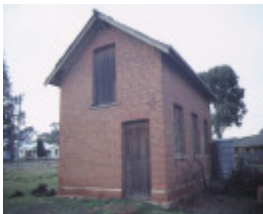
dunolly court house out building aug1984
