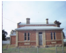
dunolly court house rear elevation aug1984
