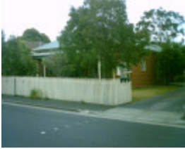
58 Albert Street Units, Geelong West
