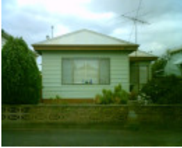
10 Avon Street, Geelong West
