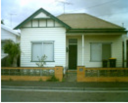
12 Avon Street, Geelong West
