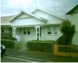
14 Avon Street, Geelong West
