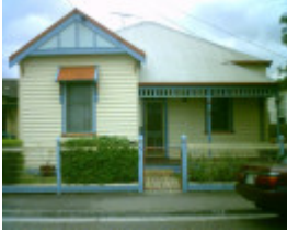
22 Avon Street, Geelong West
