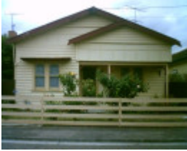
26 Avon Street, Geelong West
