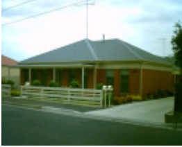
225 Hope Street, Geelong West - Units
