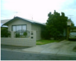
62 Clarence Street, Geelong West
