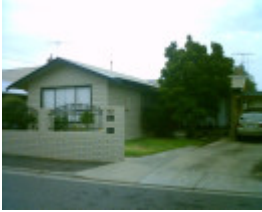
62 Clarence Street, Geelong West
