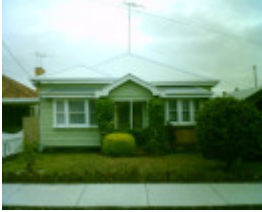
74 Clarence Street, Geelong West
