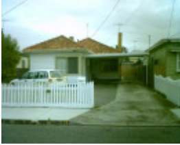
76 Clarence Street, Geelong West
