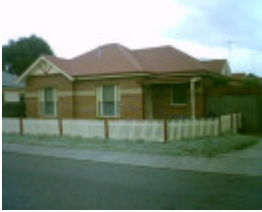
90 Clarence Street, Geelong West - Units
