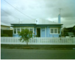
100 Clarence Street, Geelong West
