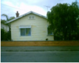
110 Clarence Street, Geelong West
