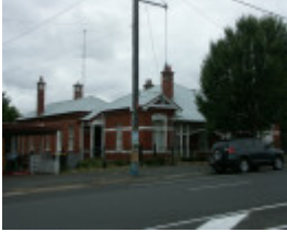
Former Bank of NSW
