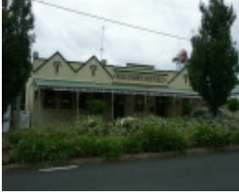
Railway Hotel (Luth's Building at Rear)
