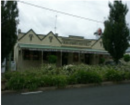
Railway Hotel (Luth's Building at Rear)
