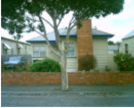
119 Clarence Street, Geelong West
